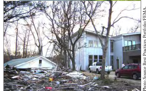
House in Bay St. Louis, MS, was built to code and survived Katrina; their neighbor's house was destroyed by Katrina.
